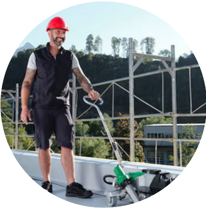
Flat Roof Waterproofing
