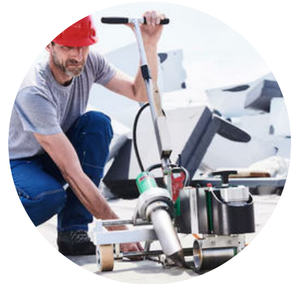
Industrial & Commercial Roofing
