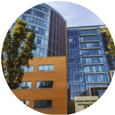
Public sector buildings
