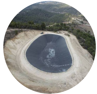
Leachate ponds cap systems
